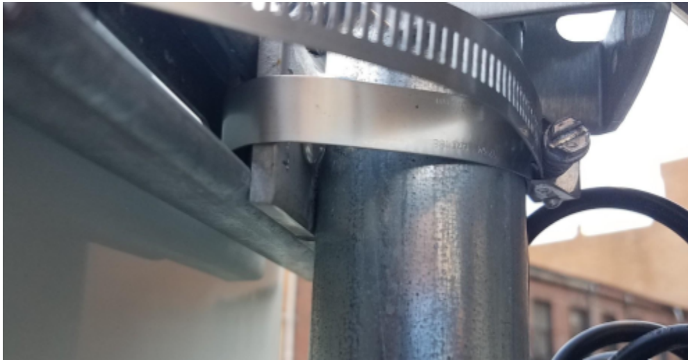
Fig 7: Close-up of panel mount
