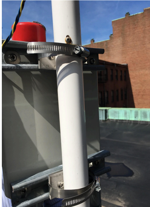
Fig 4: Hose clamps wrapping around pole to attach panel
