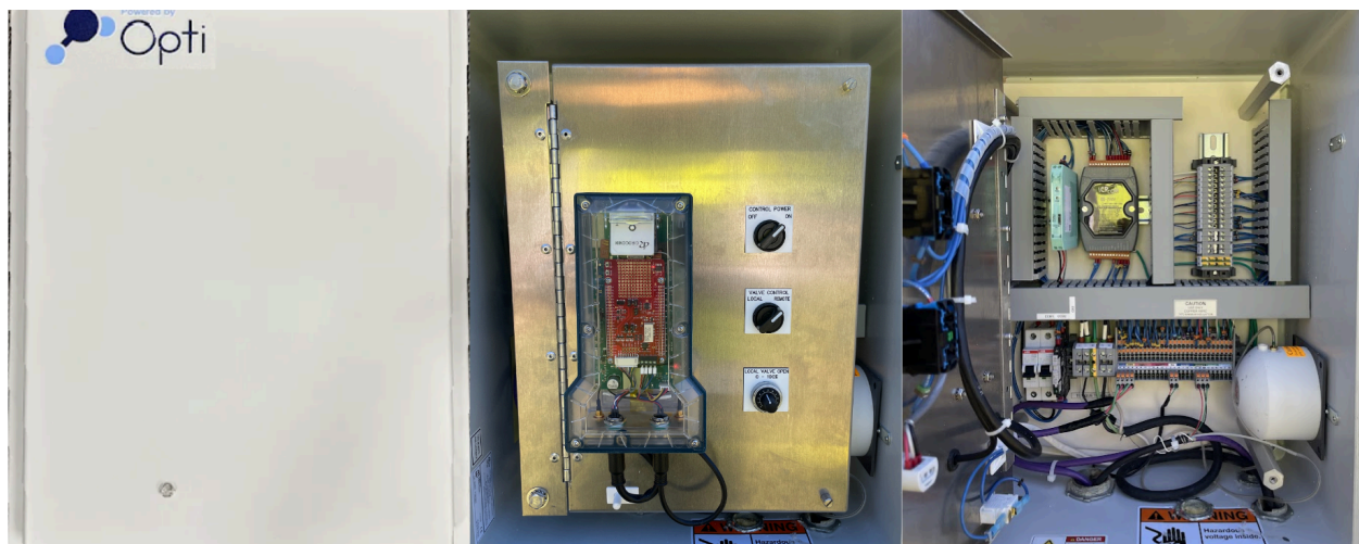
Figure 2: Opti Control Panel cover, swing door, and interior (left to right).
